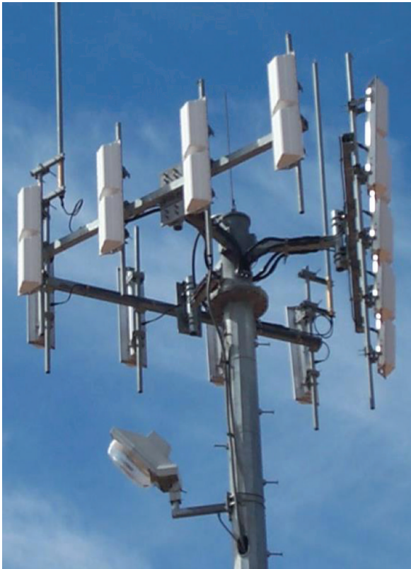
Figure 4.26 Triangular array of dipoles used as a sectoral base-station antenna for mobile communication.
